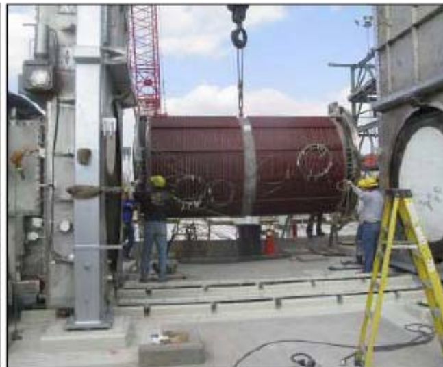
Above: MPT heating drum is inserted between the chamber doors
